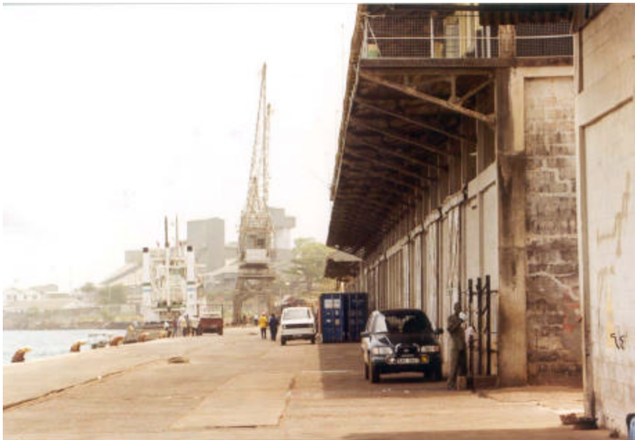
These lifting cranes were not used for years, according to port officials.
