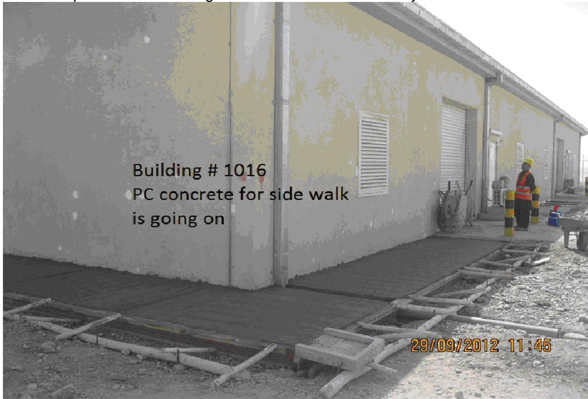
Picture 1- Sloped sidewalks being installed to divert water away from foundation.
