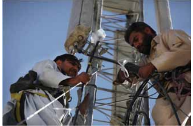
Afghan contractors working at new cellular telephone tower, Helmand province, Afghanistan (U.S. Marine Corps photo, Oct. 2010).
